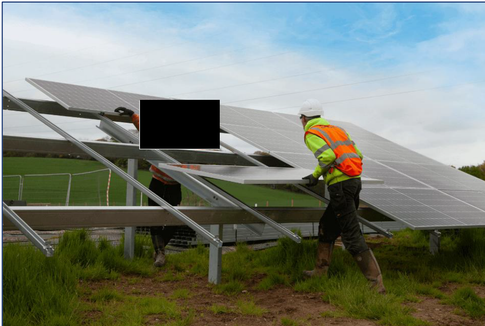
Plate 12-24 PV module installation (Ref. 12-16)
