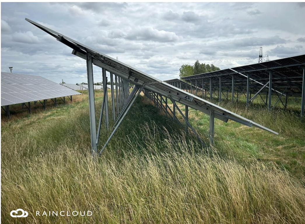
Plate 12-18 Thin PV Racking Mount
